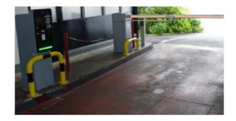
The system can be configured to open the barrier at the license place recognition. The plate is used as an identifier and no ticket is required.
